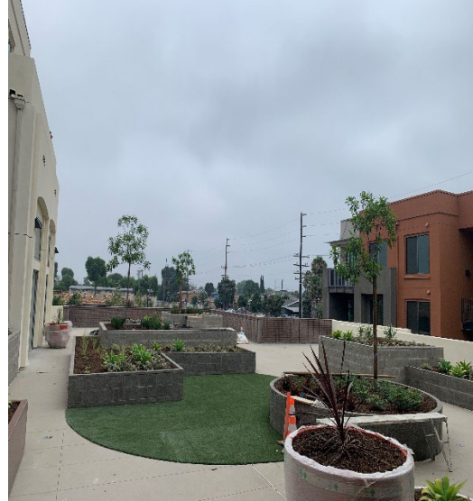
Area H2A - View of Podium building exterior courtyard June 13 ,2024
