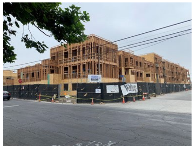
Area S4 – Construction in progress
