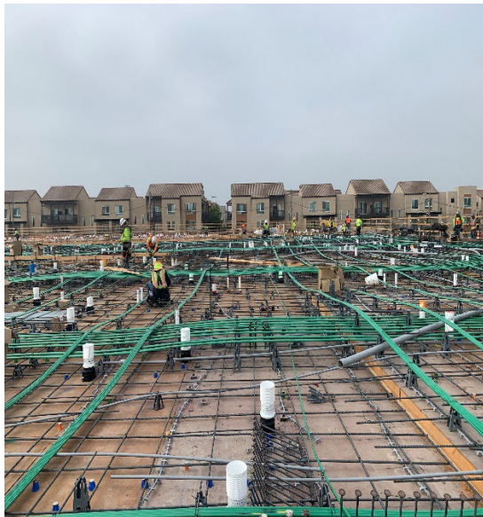
Area H2B – Podium building PT deck June 6, 2024
