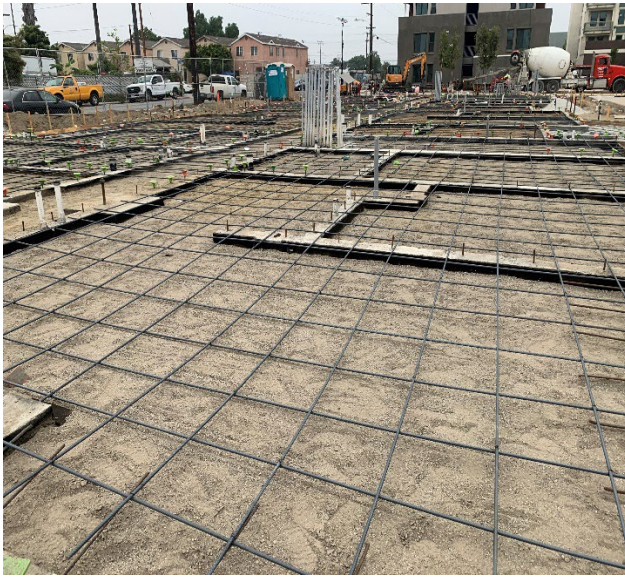
Area H2B – View of 2 story building slab on grade June 13, 2024
