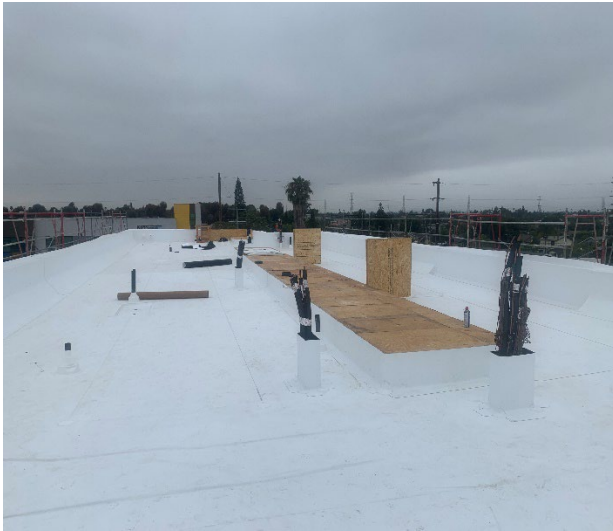
Area S4 – View of building A roof June 12, 2024
