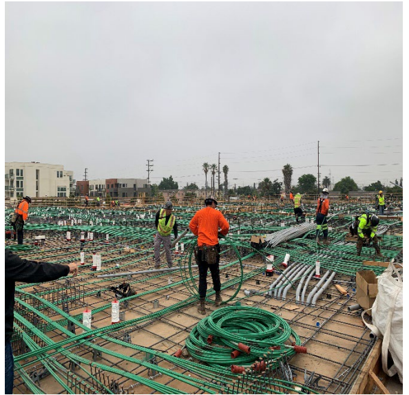
Area H2B – Podium building PT deck June 13, 2024
