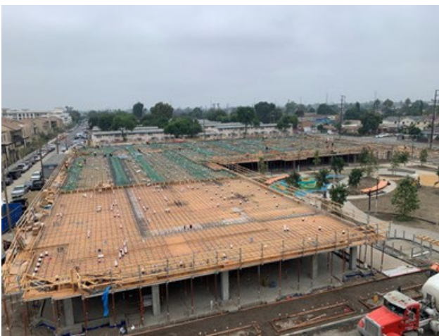
Area H2B – Construction in progress
