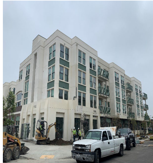
Area H2A - View Podium building exterior June 13, 2024
