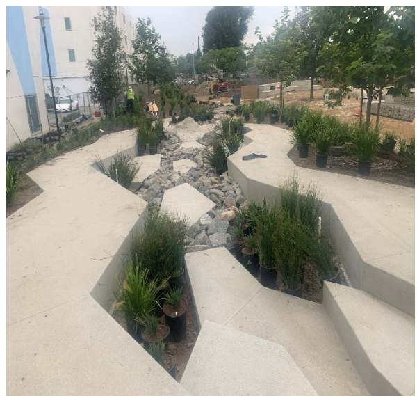
Area FTP – View of site June 12, 2024
