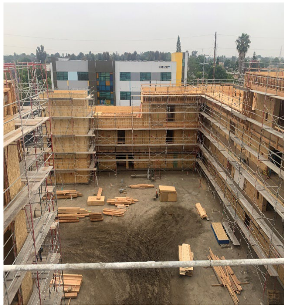
Area S4 – View of building A May 22, 2024
