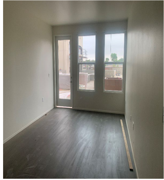
Area H2A - View of podium building unit May 16, 2024
