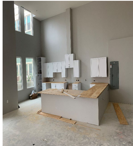
Area H2A - View of Podium building community room June 13, 2024
