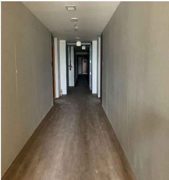
Area H2A - View Podium building corridor flooring June 13, 2024
