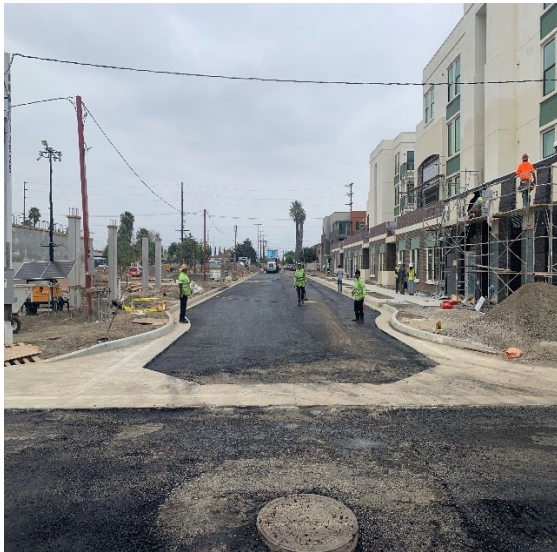
Area H2A – View Kalmia st paving unit May 2, 2024
