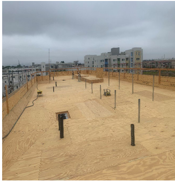
Area S4 – View of site building B roof June 12, 2024
