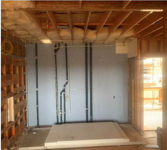
Area S4 – View of building A nit June 12, 2024
