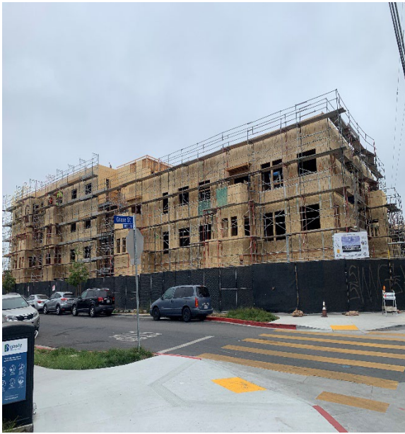
Area S4 – View of building A framing May 29, 2024
