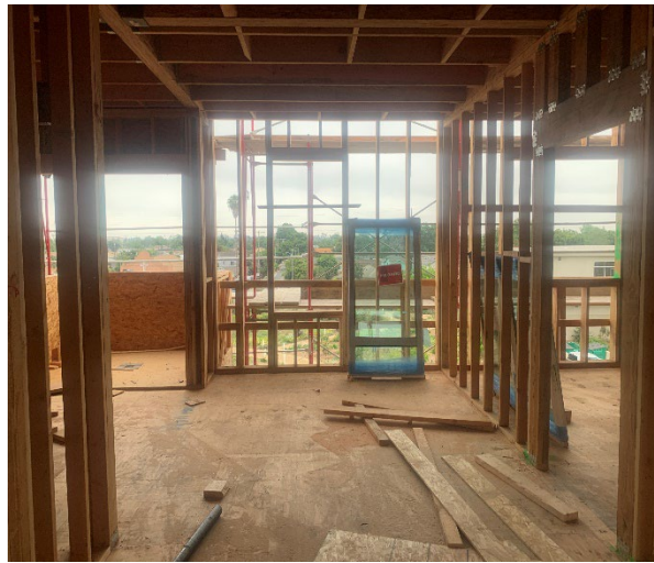
Area S4 – View of building B unit June 12, 2024
