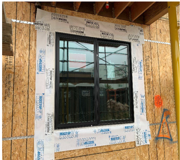
Area S4 – View of building A windows June 12, 2024
