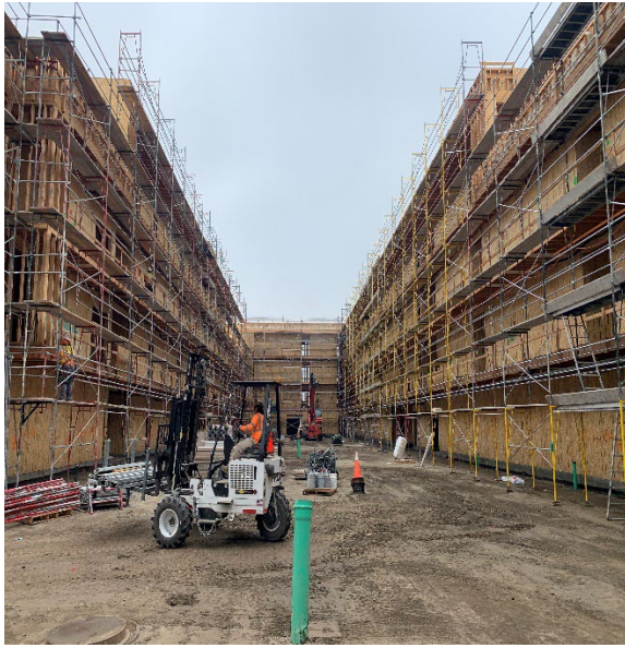
Area S4 – View of building B June 12, 2024
