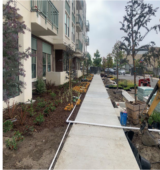
Area H2A - View of Podium building landscaping June 6, 2024
