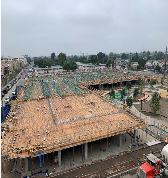
Area H2B – Site picture June 13, 2024
