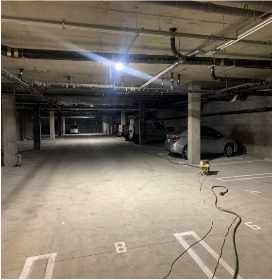
Area H2A - View of Podium building garage June 6, 2024
