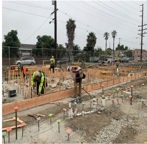
Area SH2B - View of 3 story building footing and stem walls June 13, 2024
