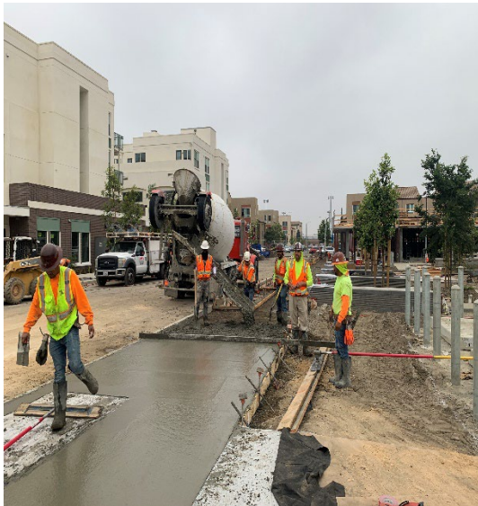
Area H2A - View of Kalmia st sidewalk June 13, 2024
