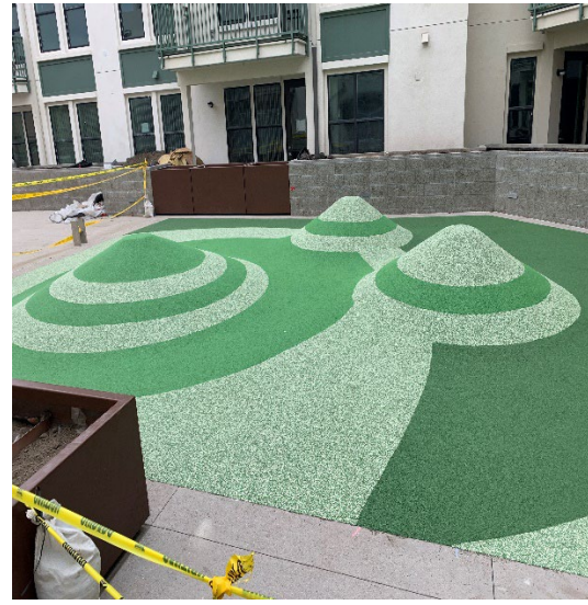
Area H2A - Podium building courtyard play area May 9 , 2024
