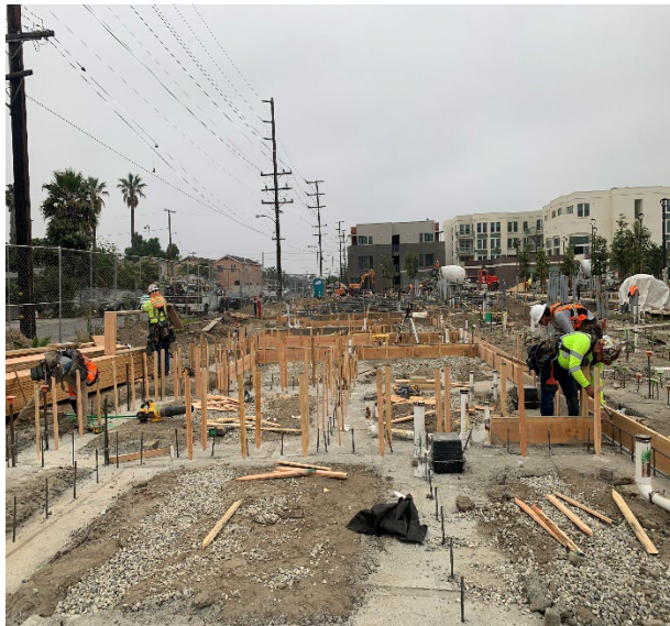
Area SH2B – View of 3 story building footings and stem walls June 13, 2024
