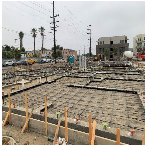
Area H2B – View of 2 story building slab on grade June 13, 2024
